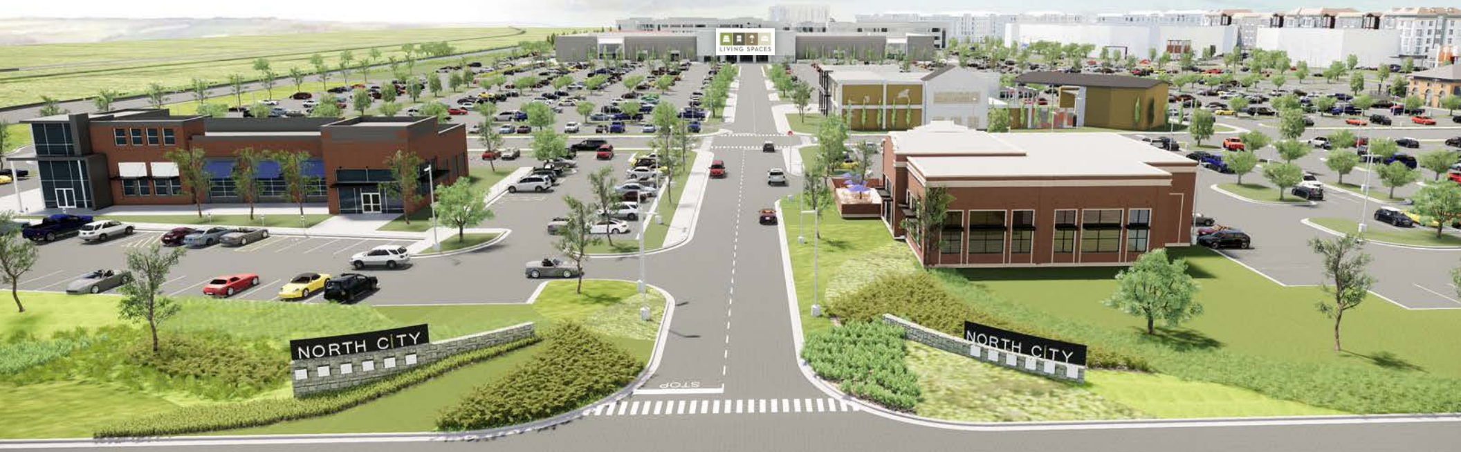
Looking South at The Omni building
